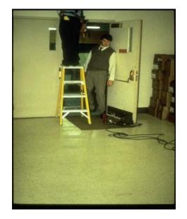
Ladders not placed in front of doors opening toward the ladder unless the door is blocked upon, locked, or guarded;
